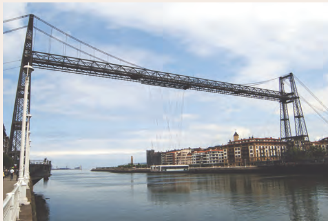
Vizcaya Bridge (Spain)
